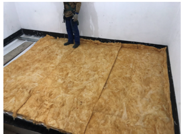
Figure 10: Installation of the glass wool.
