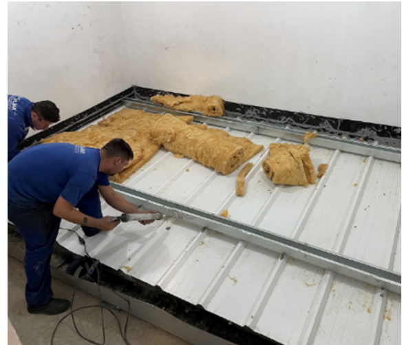
Figure 8: Installation of the roofing system in the chamber.
