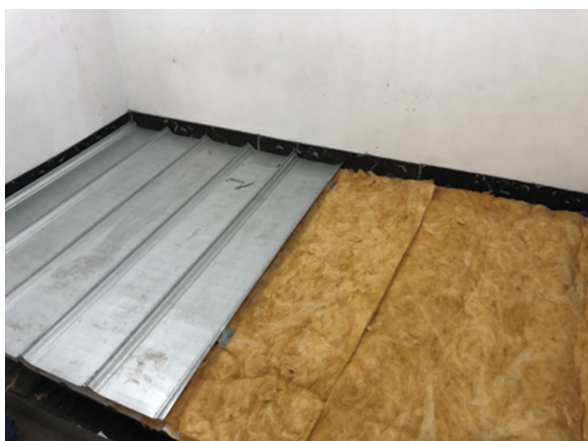
Figure 11: Installation of the upper zipper roof tile.
