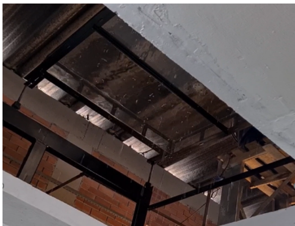
Figure 5: Internal view of Water Tank 1 with the perforated plate.
